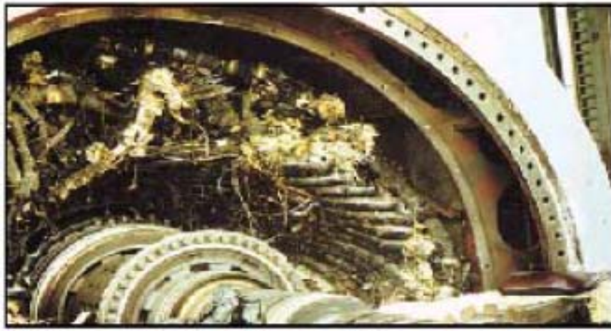
Figure 7: Consequences of a failure in a retaining ring
