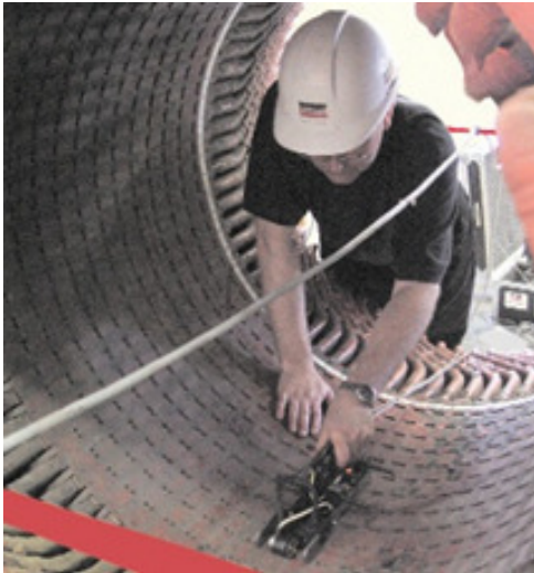
Fig B8-3: During Stator core low energy test
